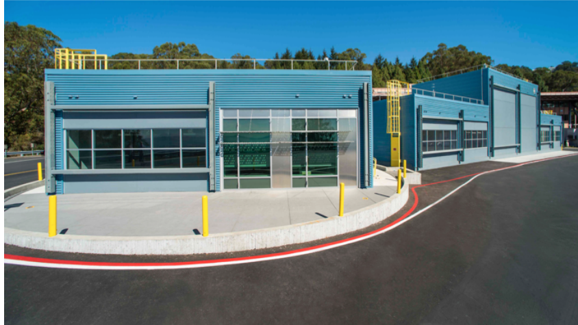
Figure 1. LBNL's FLEXLAB, A Commercial Integrated Systems Test Facility
